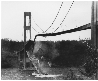
(a) Tacoma Narrows Bridge Collapse (Encyclopaedia Britannica, 1940)
