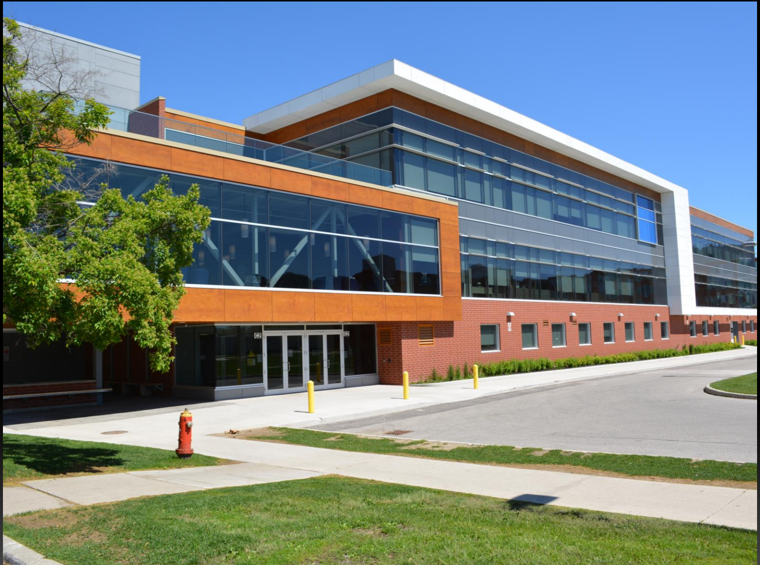
Newly Constructed Engineering Building
