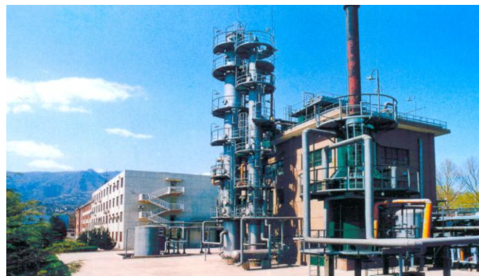
Figure 4. Hydroisomerization Unit at Yanshan Petrochemical
