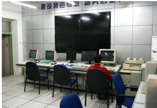
Figure 5. On-Campus Control Room of Experimental Platform
